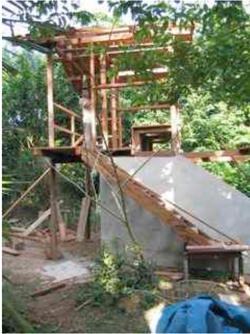
Building a Ferro-Cement Composting Toilet
